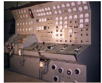
Panels after restoration
